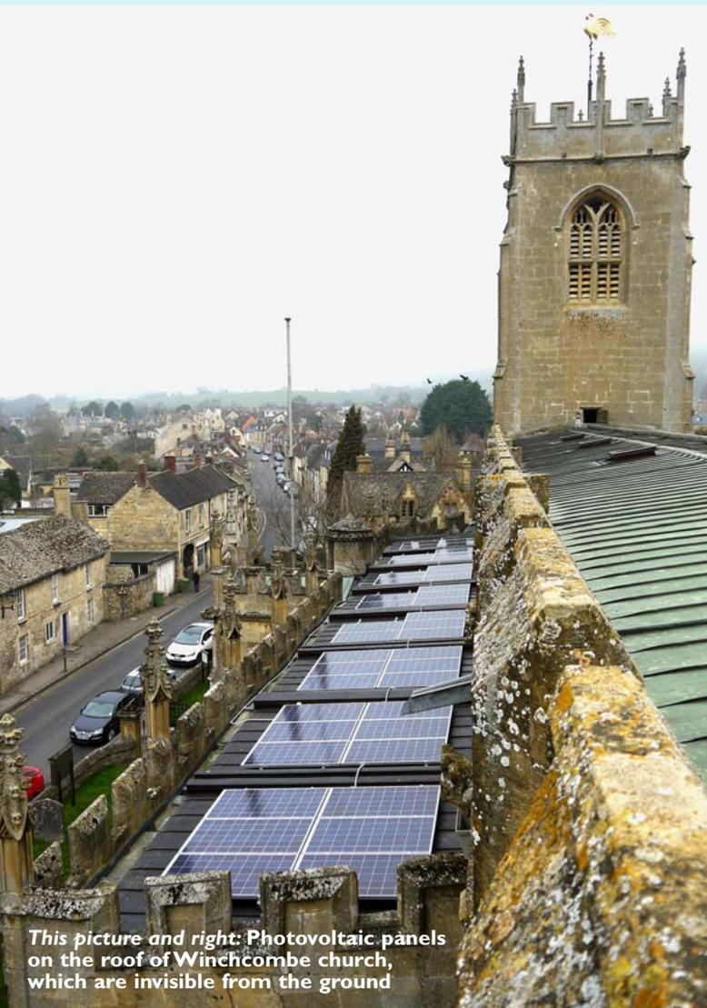
*This picture and right: Photovoltaic panels on the roof of Winchcombe church, which are invisible from the ground*
