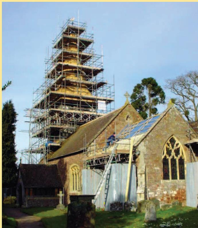
**Right: Work in progress at St Mary the Virgin, Bromesberrow to re-shingle the spire with cleft oak shingles and re-roof the chancel in stone slate**
