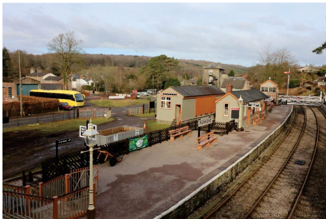
Parkend Railway Station
